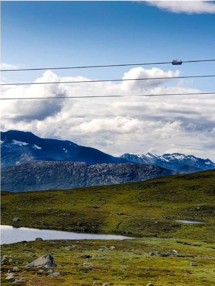
The TLM monitor measures conductor sag via inclination and uses built-in LiDAR to directly measure the distance from the conductor to the ground below.
